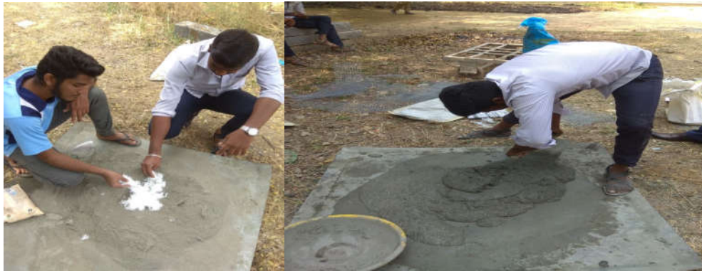
Fig 2. Adding and Mixing of concrete
